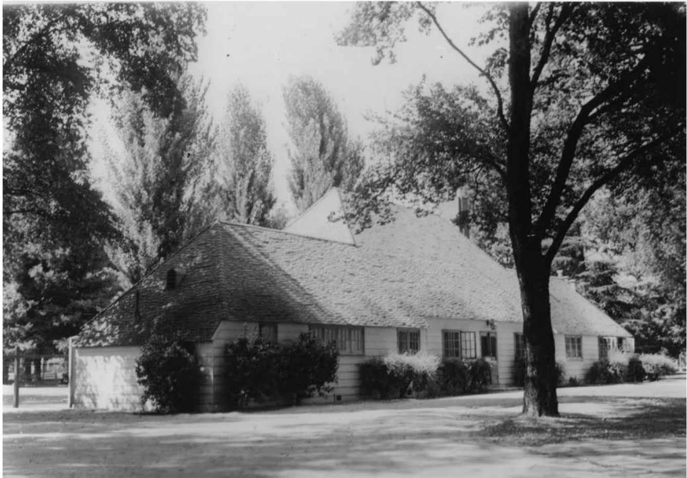
Figure 10, Southside Park clubhouse, no longer extant. Sacramento Public Library photo
